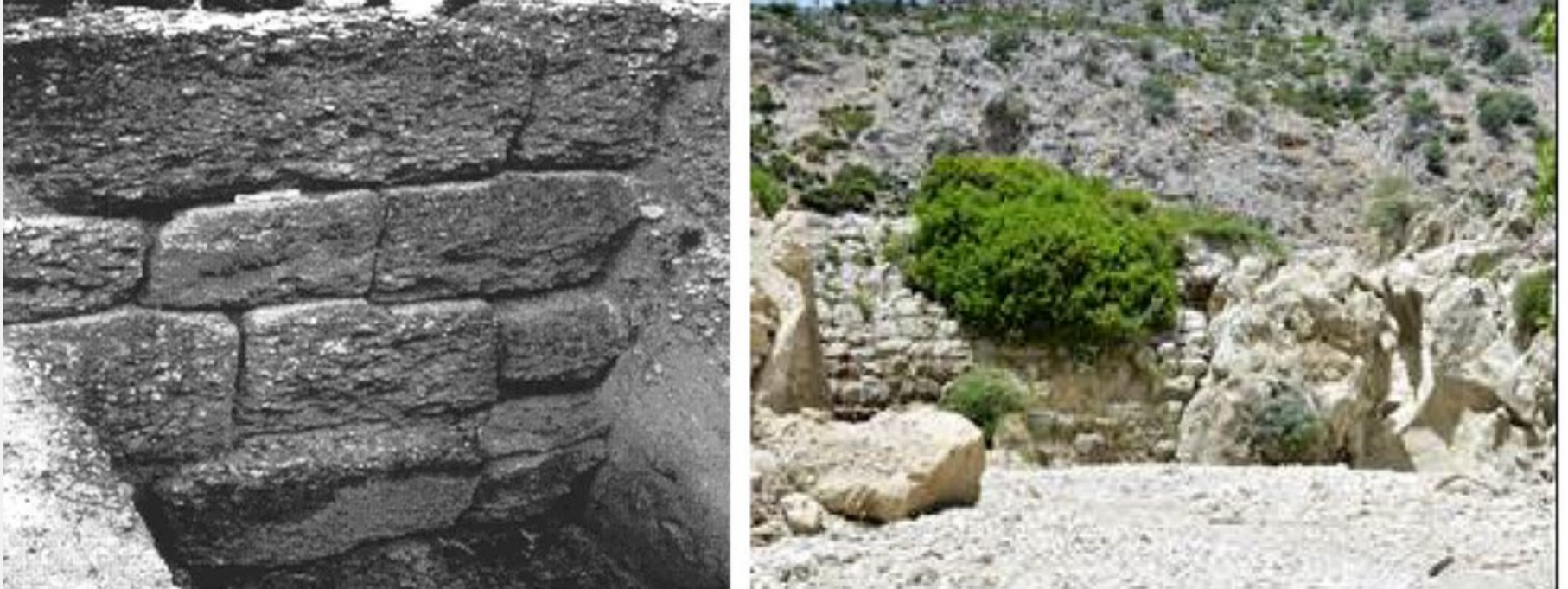
Fig.7 Stream control hydraulic works in ancient Greece: a the wall blocks of Kladeos stream in ancient Olympia (Koutsoyiannis et al. 2008) and b the dam of Alyzia (Photograph A. N. Angelakis)
